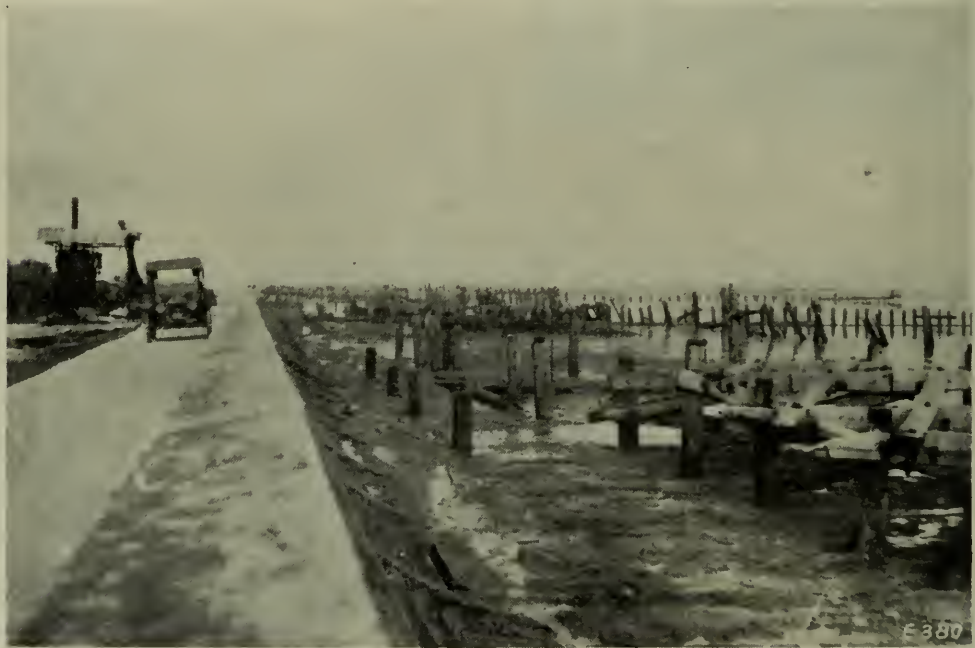
FIG. 1. SEA WALL ON EAST COAST SHOWING ABANDONED WOODEN PROTECTIVE WORKS.
